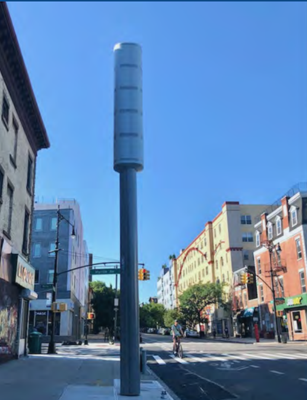
New York City Jumbo 5G poles with 5 tiers to house transmitting antennas from numerous carriers.
