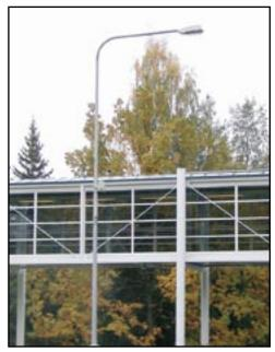
Base station integrated into lightpole
