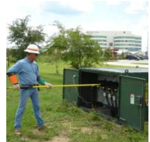
A 3-phase SF6 switch used in electrical utility distribution.
