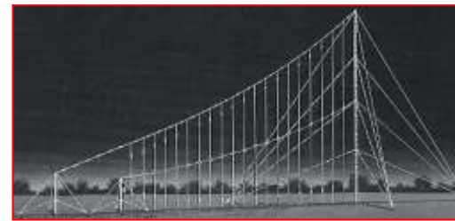
The figure shows an array of dipoles of various lengths used for broadcasting. The waves are vertically polarized.
