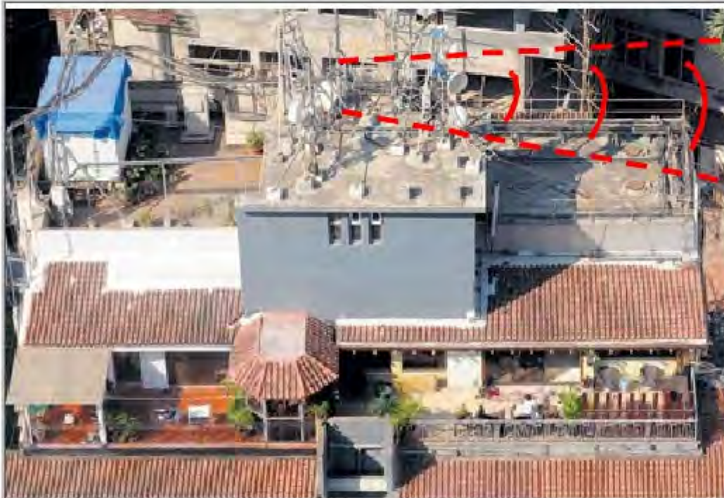
The cell phone towers installed on the Vijay Apartments terrace at Carmichael Road pic/Bipin Kokate
